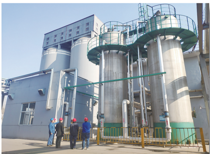
钢铁行业焦化废水深度处理现场调研
