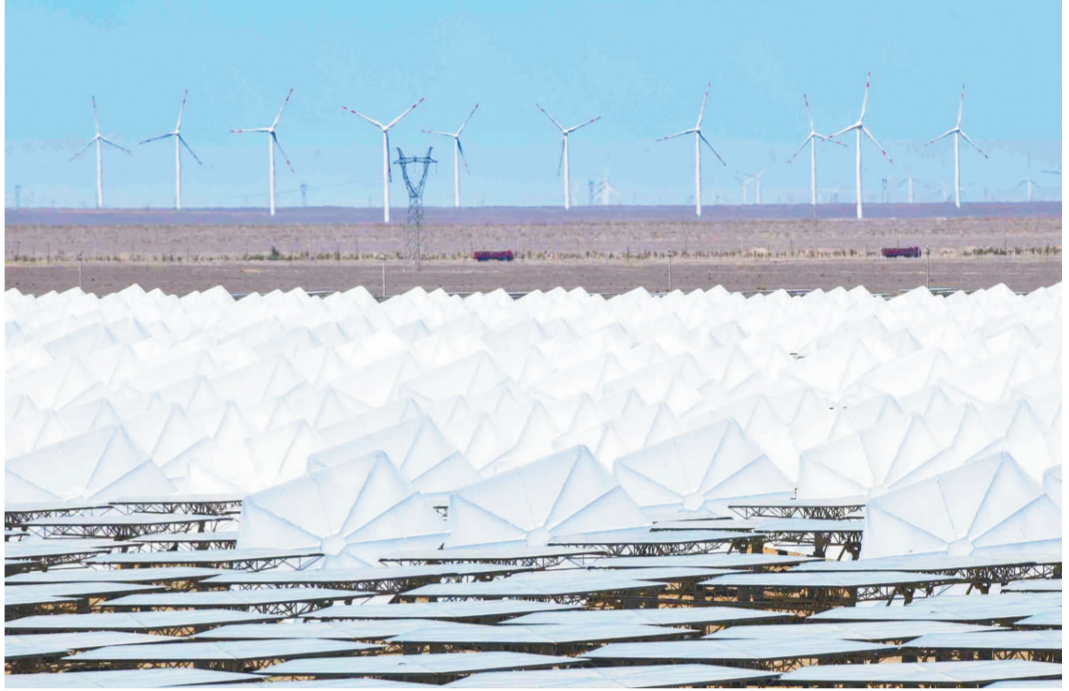
图为哈密塔式50兆瓦光热发电站局部场景。李华摄
